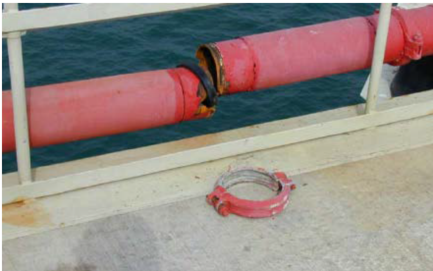
Figure B.6-4 – Support break. Peru 2001 M 8.4.
