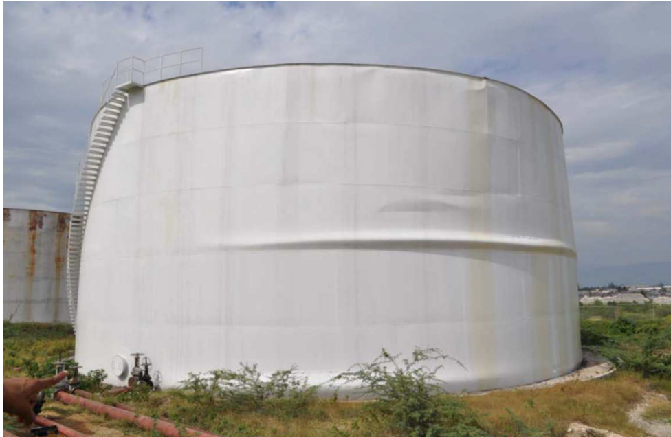
Figure B.5-5 – Elephants's knee and foot buckling. Haiti earthquake in 2010, M 7.0.
