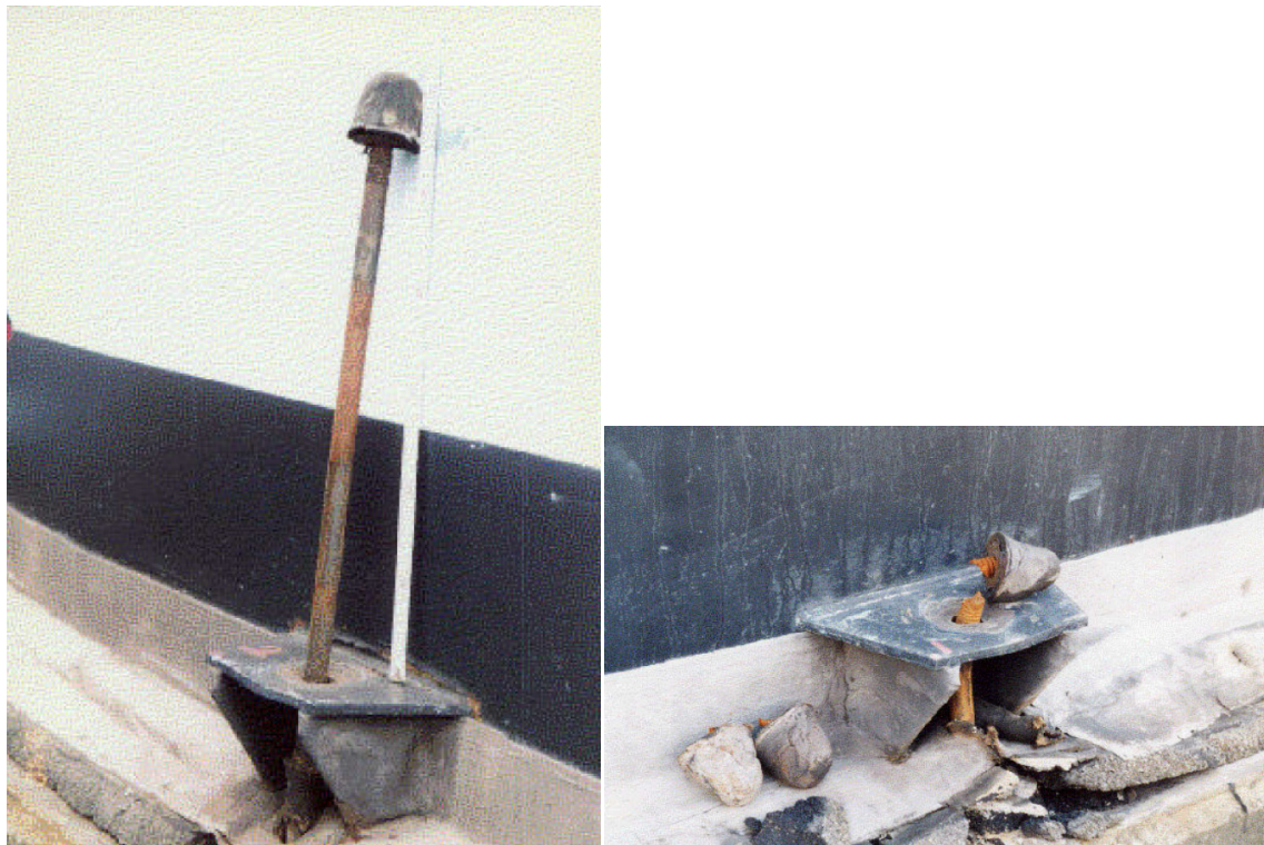
Figure B.5-10 – Damage and rupture of anchorages. Kobe (Japan) earthquake 1995, M 7.3.
