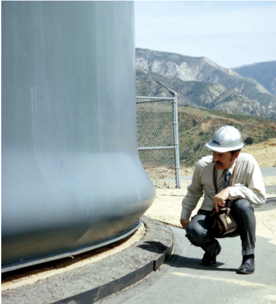
Figure B.5-3 – Elephants’s foot buckling. San Fernando earthquake in 1971, M 6.6.
