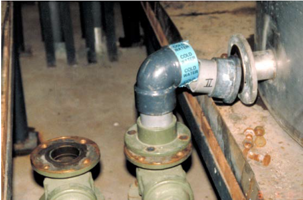
Figure B.6-1 – Pipe elbow failure at the base of a water tank. Edgecumbe (New Zealand) 1987, M 6.3.
